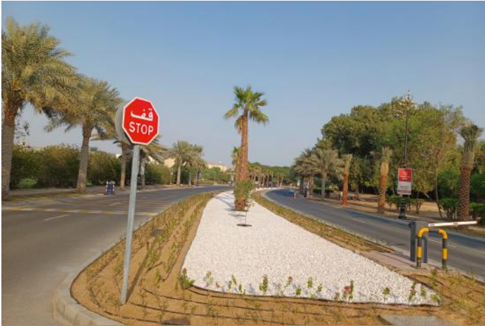
Gate 1 & 2 areas – Centre median planting works in progress
