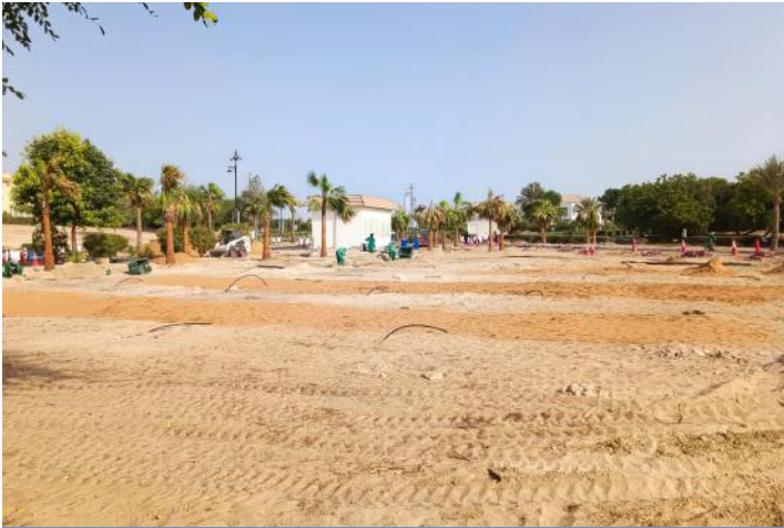
Area between Clusters 26 & 27 – landscaping enhancement preparation works completed.
