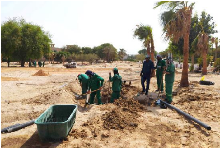
Area between Clusters 26 & 27 – irrigation and tree planting preparation works completed.
