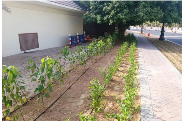
Gate 1 & 2 areas – right-of-way planting works in progress
