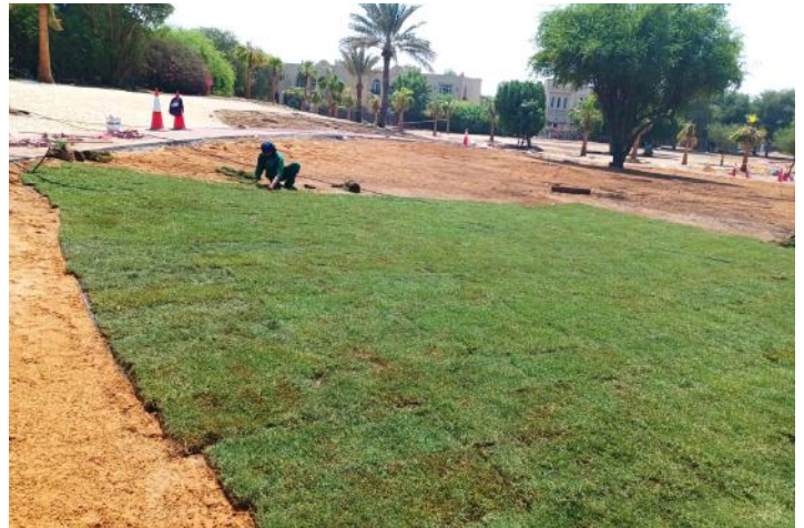
Area between Clusters 26 & 27 – landscaping enhancement works in progress.
