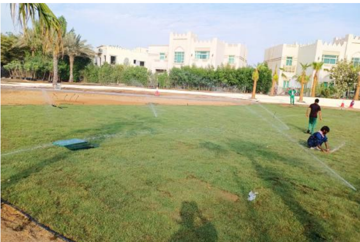
Area between Clusters 26 & 27 – irrigation and grass planting works completed.
