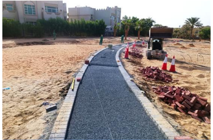
Area between Clusters 26 & 27 – additional footpath installation in progress.
